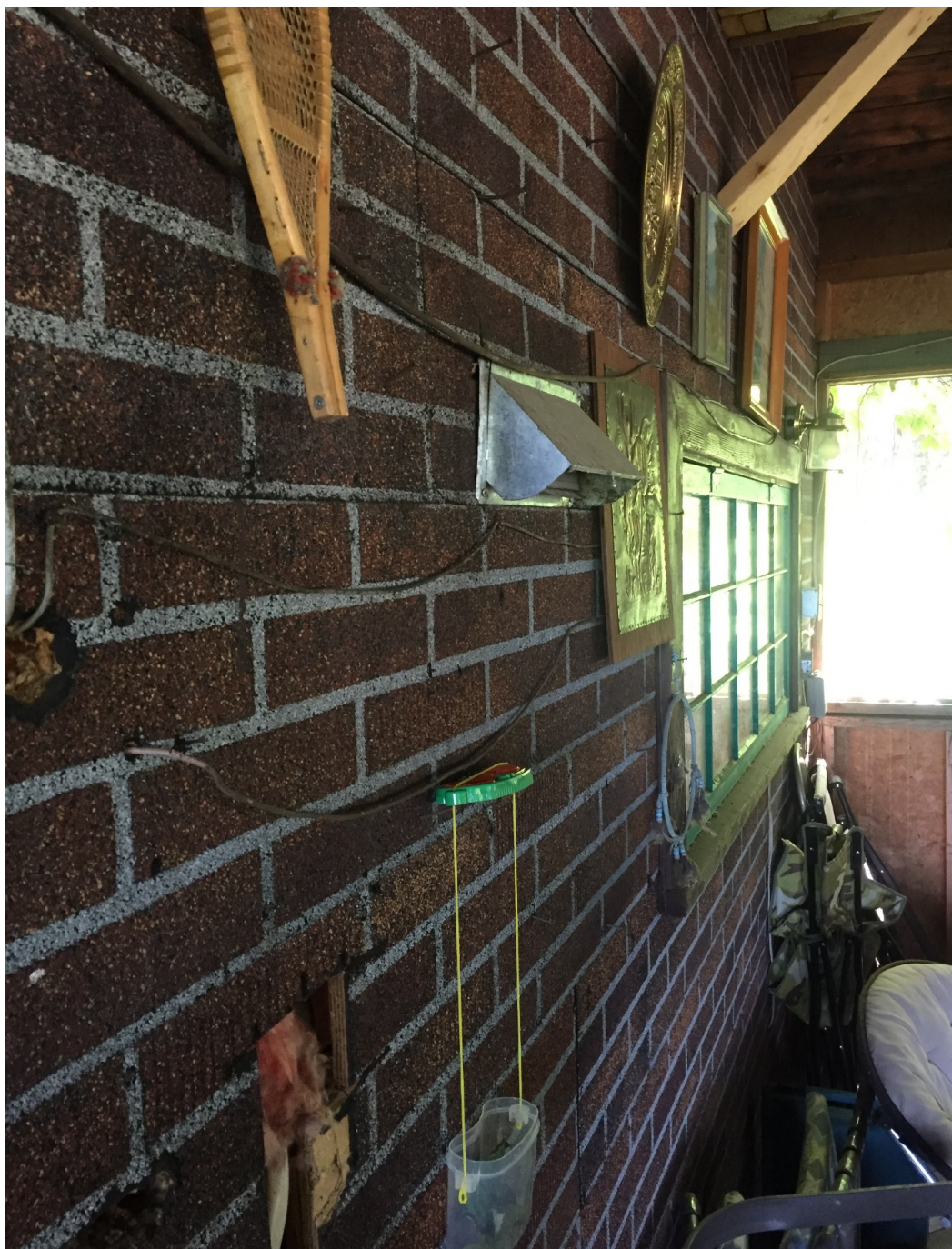
Figure 3 Photo from 2018 site visit: Front porch of 1338 Thompson Rd., exposed wiring and Insulbrick siding
